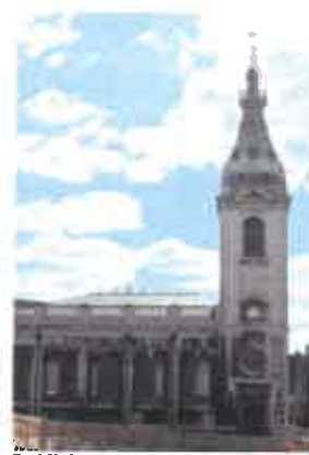
St Nicholas as restored in 1962, viewed from the north in 2016
